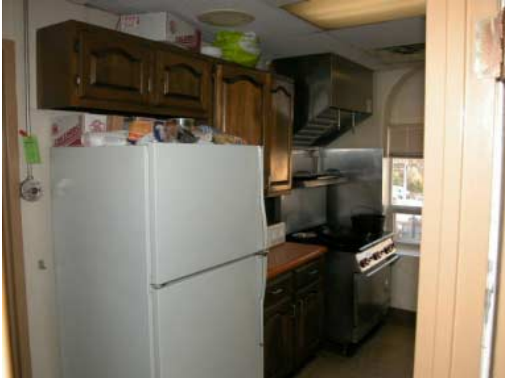
Figure 12 Station 5 View of the south wall of the kitchen
