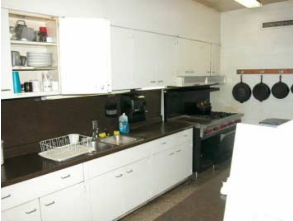
Figure 17 Station 27 View of the west kitchen wall and the north corner
