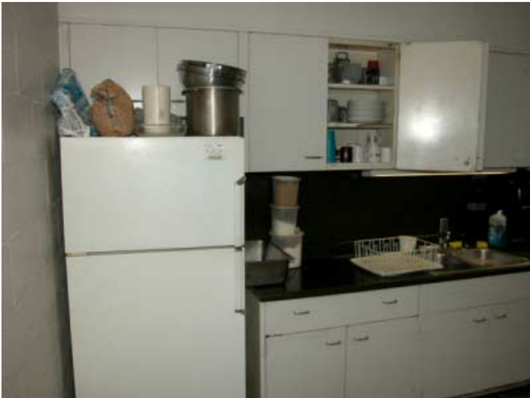
Figure 16 Station 27 View of the south corner of the west kitchen wall
