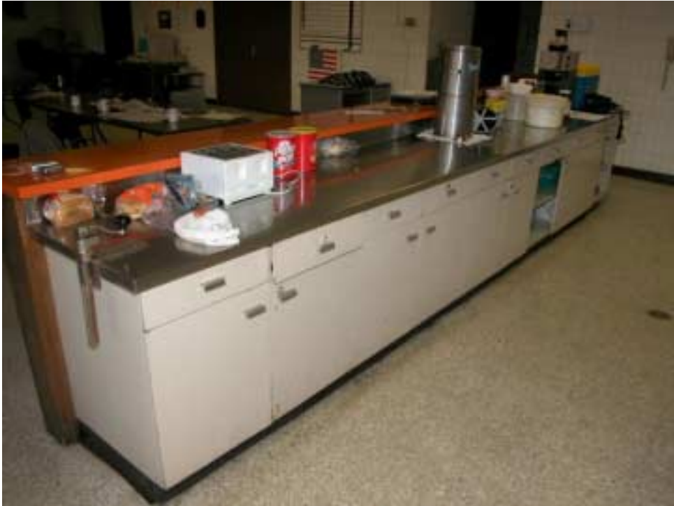
Figure 6 Station 4 The island cabinets will be replaced. The countertop should be re-used if possible.
