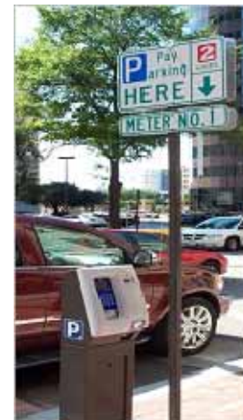
The City of Tulsa recently installed centralized, multi-space on-street pay stations with clearly defined signs to help increase the ease of use and overall utilization of on-street parking.
